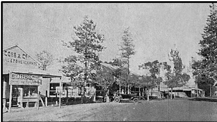
Looking down Pine Street from near the Park, 1924 (SLQ).
