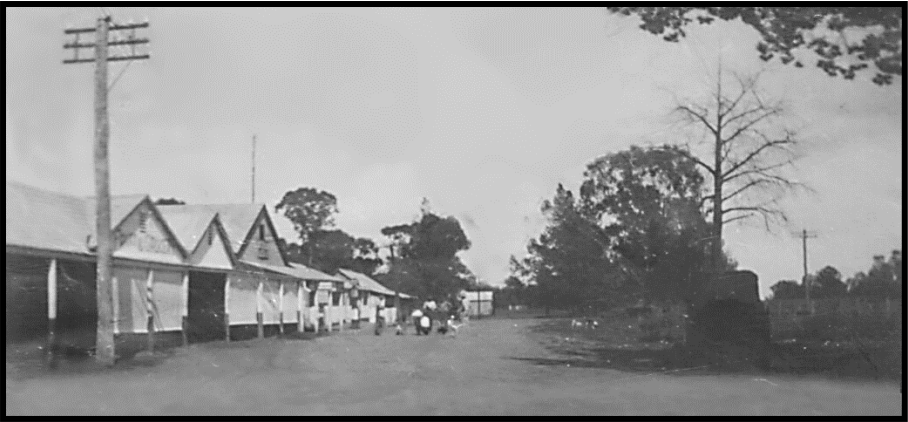
(Above) Looking west along Pine Street from Booligar Street.
