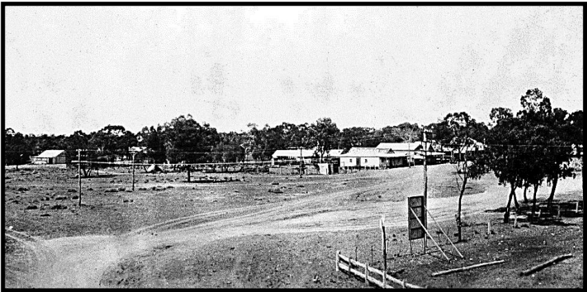
View from the railway crossing, across Pine Street to Garah Street, early 1930s. Site of the Park at front right, the former Cobb & Co store and stables in centre and the former Deeley's garage on left in distance (NAA J2879, QTH295/16).
